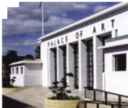
The Palace of Art in Glasgow uses external wall insulation.
