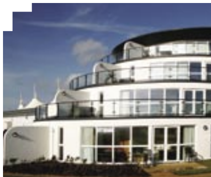
The Shoreline Hotel, Bognor Regis uses external wall panels.
